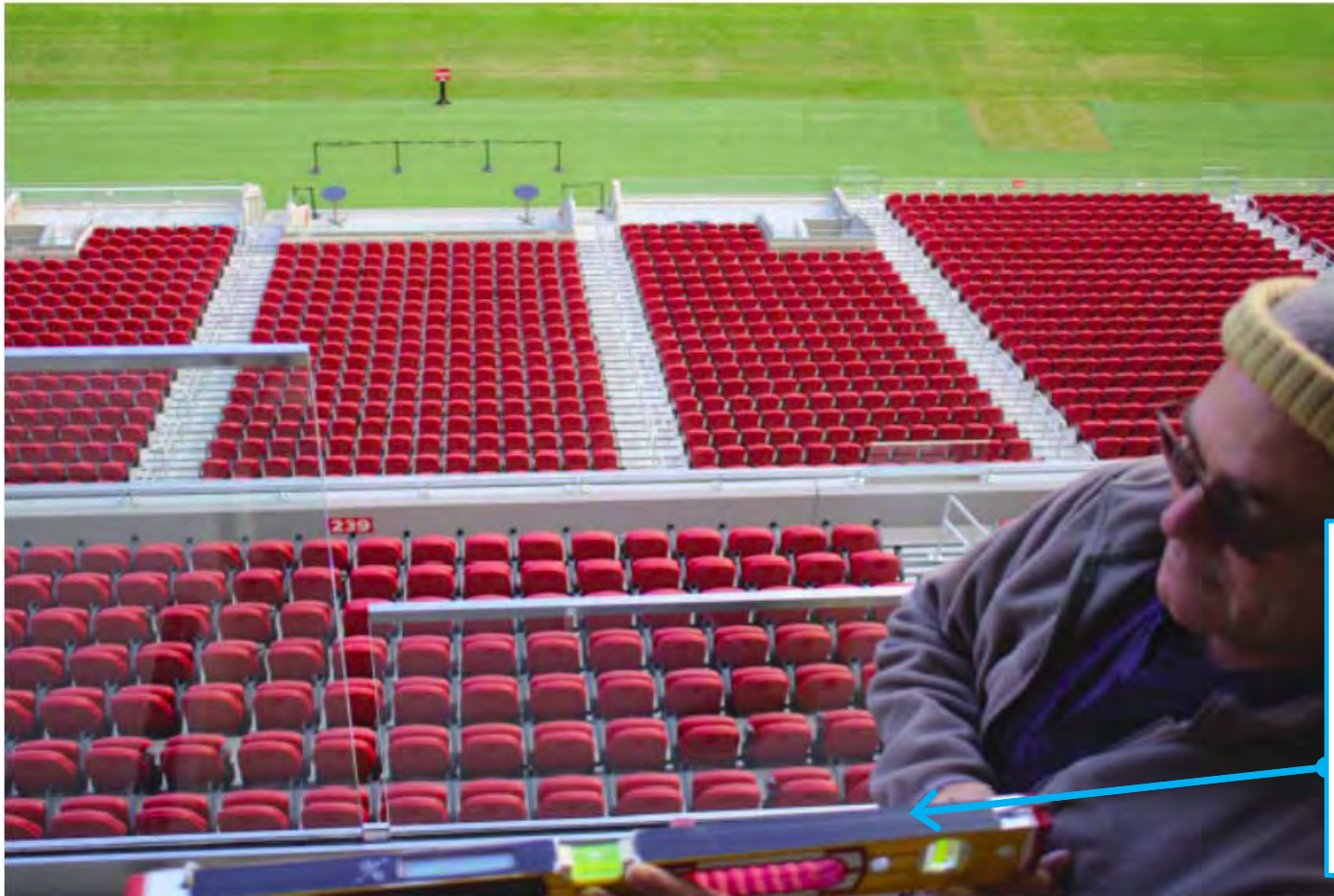
FAVORABLE VIEW LUXURY SUITE SIGHTLINE FROM WHEELCHAIR ACCESSIBLE SEAT Vantage point: eye height of a standing spectator = 63.45" AFF
